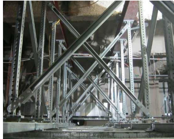
Figure 1. 1 Cross Bracings
